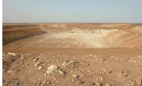
縦75m横60m深さ4mの貯水池を掘削
